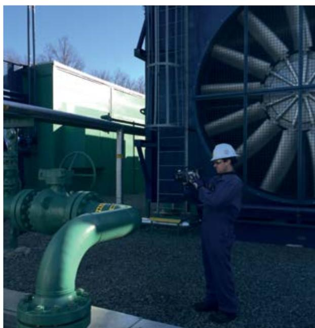
Operator conducting leak detection and repair survey with an optical gas imaging (OGI) camera on one of our Appalachia sites in the USA.
