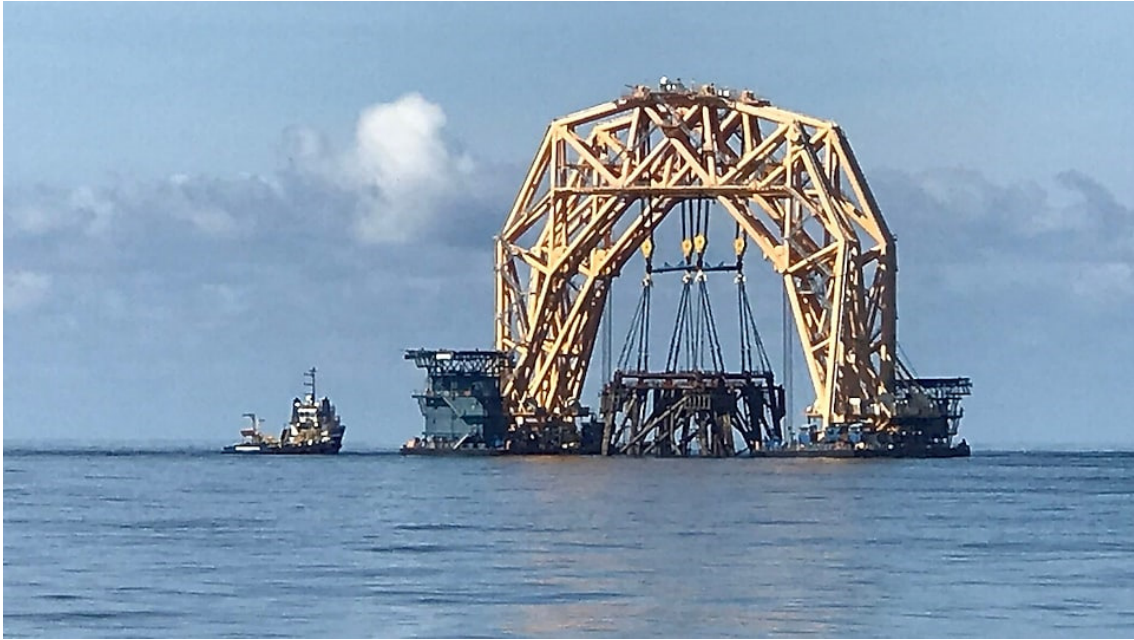
Cougar's jacket travelled on a nearly 50 mile open water journey to its new home
