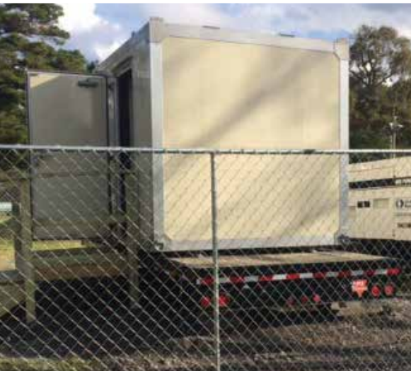
An EPA and DEQ Sulfur dioxide monitor is housed within a small building behind the former Bill’s Dollar Store. The SO 2 monitoring project represents a cooperative program among seven area industries.
